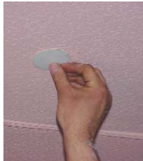
Plugging the ceiling hole
