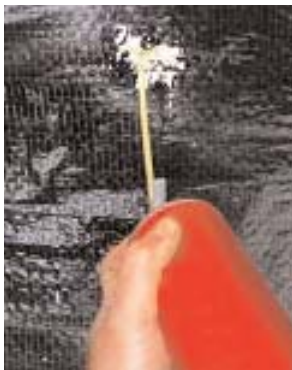
Using foam sealant on the bottom board
