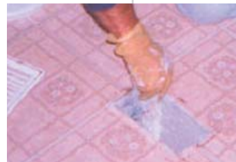
Sealing around a register with duct mastic
