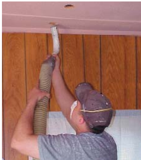
Blowing insulation through the ceiling
