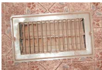
Floor register with louvers closed
