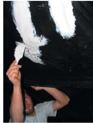
Using mastic to seal a bottom board patch
