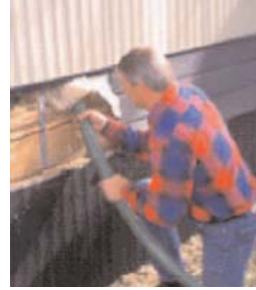
Blowing wall insulation
