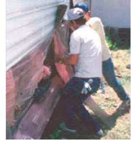
Stuffing fiberglass batts into a sidewall
