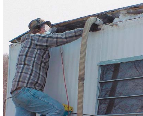
Blowing insulation into the roof
