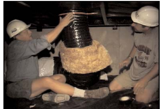
Fastening the inner lining of the crossover duct to the collar
