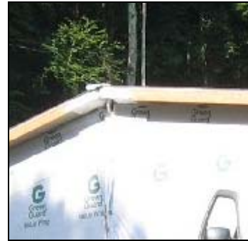
Fascia boards at gable end
