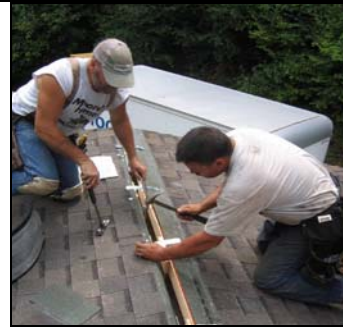
Installing straps across ridge gap
