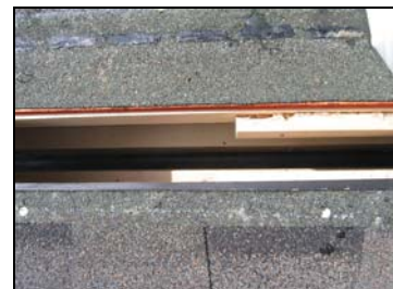
Shingles extend fully to ridgeline
