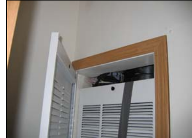
Furnace closet clearance
